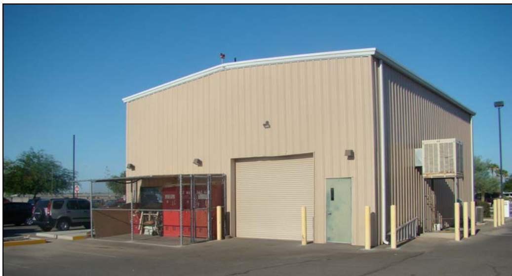
Source: Yuma International Airport, August 2008. Prepared by: Ricondo & Associates, Inc., August 2008.
